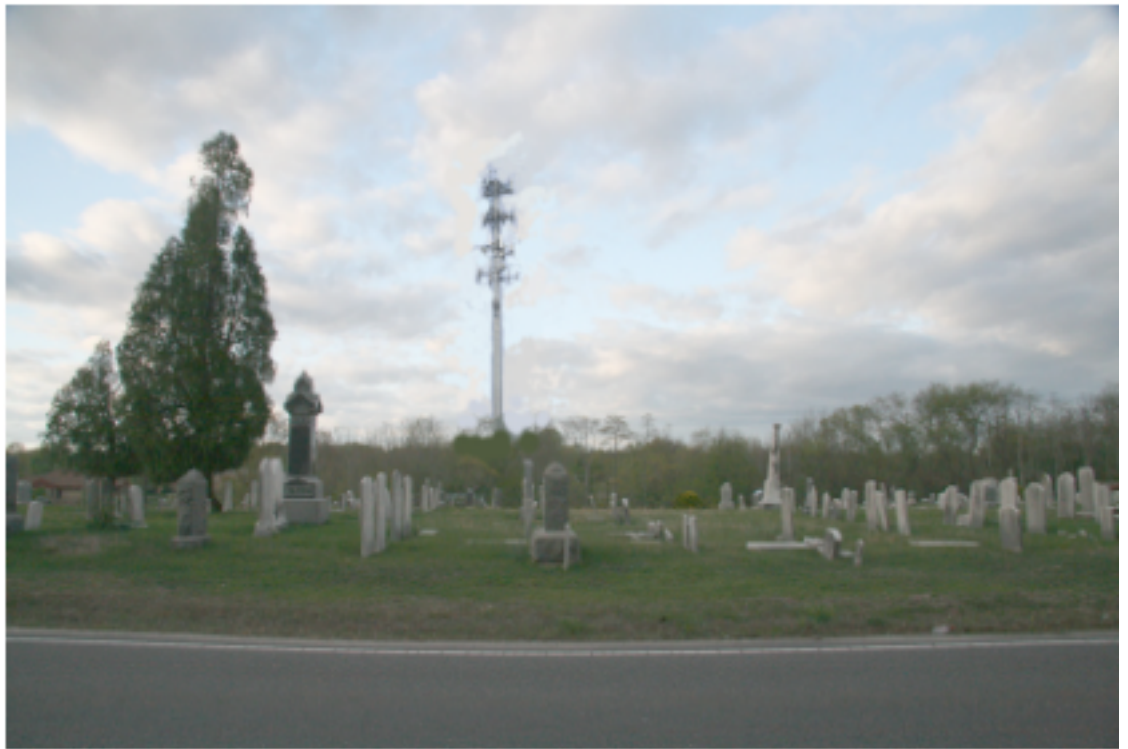
VIEW OF PROPOSED CELL TOWER FROM OLD CORLIES AVENUE JUST EAST OF WEST BANGS AVENUE (Church Hill) AND HAMILTON UNITED METHODIST CHURCH
